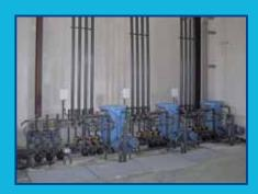
probe for pH and conductivity. • Total control depending on the demands or preferences of the customer, with control of the time and volume of injection, desired/increased EC, desired acidic or basic pH, with independent control of proportional volume for each injector. • Totally automated with control from the electric panel or a remotely connected PC.
